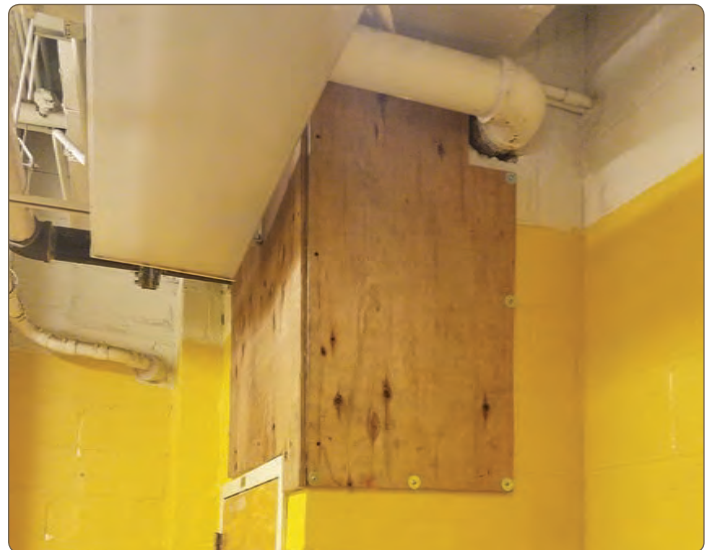
This hole was repaired to make the infrastructure complete.
