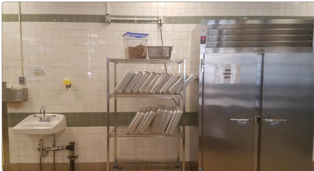
Installation of new handwashing sink and electrical for new raw protein reach-in refrigerator.
